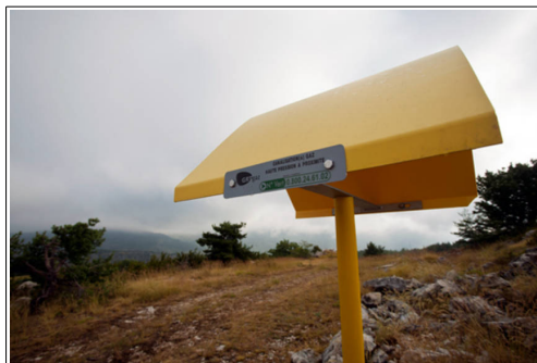
Balise (Source : GRTgaz)
